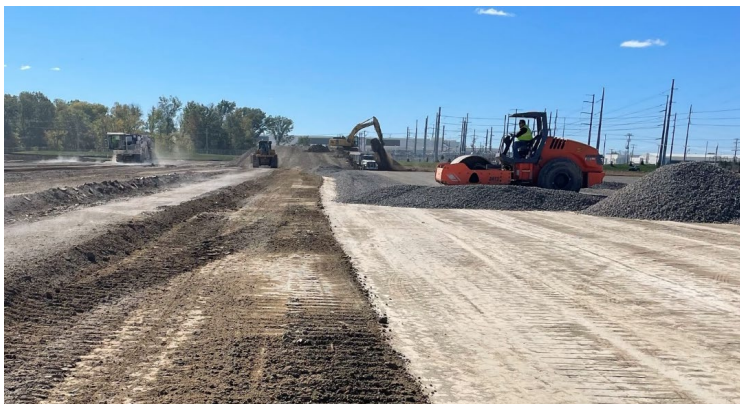
Figure 7. Stone Application Immediately Following CQL addition, mixing and compacting.
