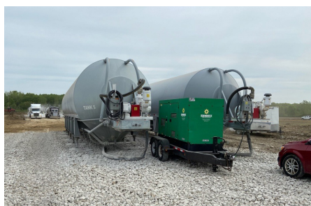
Two PIGS with electric blowers and an onsite generator
