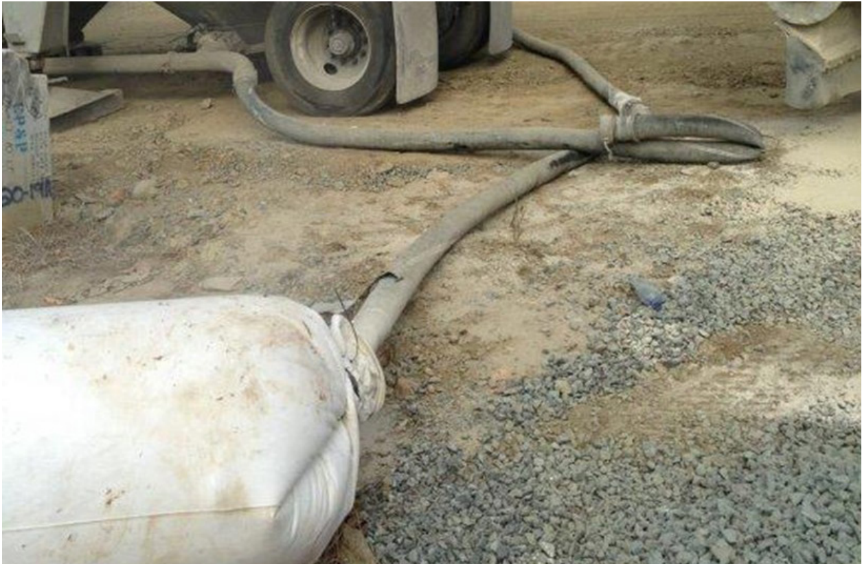
FIGURE 4. PICTURE OF VENT PIPE CONNECTED TO A FILTER SOCK
