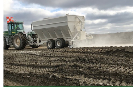
TRACTOR TRAILER WITH SPREADER BEING USED SPREAD QUICKLIME
