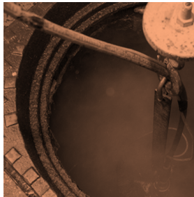
Pipe & Drain Cleaning
