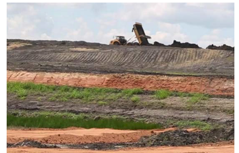
CALCIMENT LKD IS APPLIED TO STABILIZE THE UNDERLYING SUB - BASE
