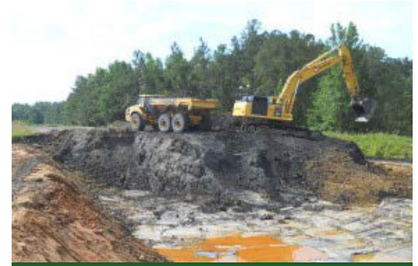
COAL ASH HOLDING BASIN EXCAVATION
