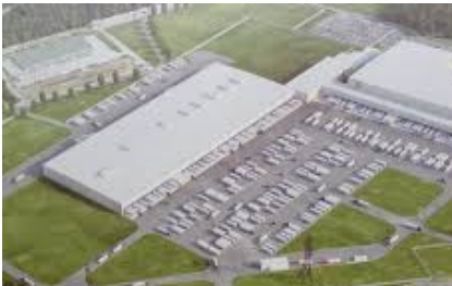
KROGER DISTRIBUTION CENTER - GA
