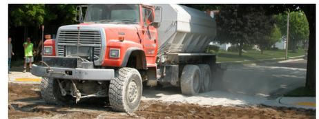
FDR & SOIL STABILIZATION WITH CALCIMENT REBUILDS XENIA STREETS
