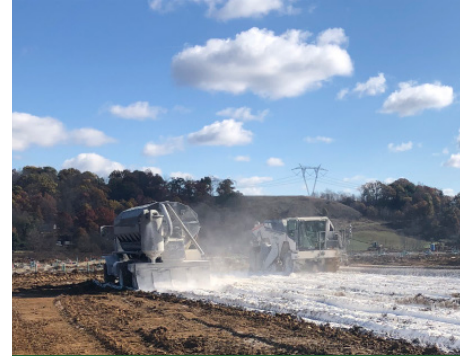
Spreading Quicklime & Mixing With Reclaimer
