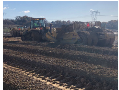
Moving Treated Soil to Fill Location
