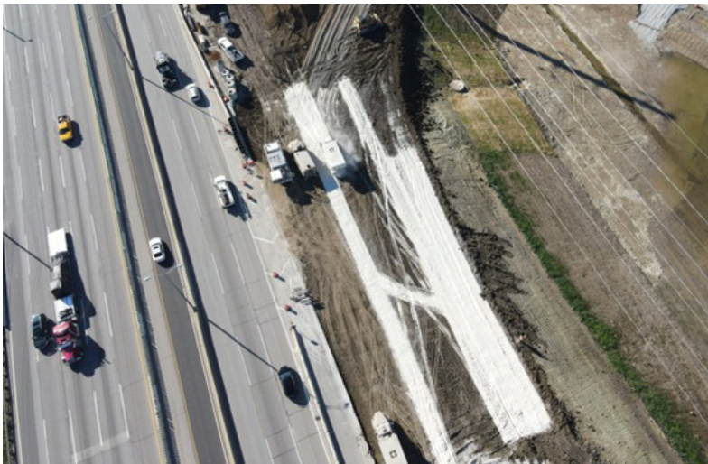
Aerial view of the I-294 job
