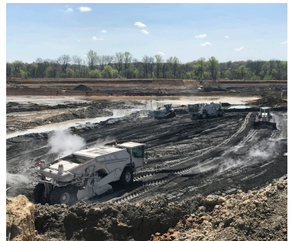
Lime Fines being mixed into the Ash with a Reclaimer
