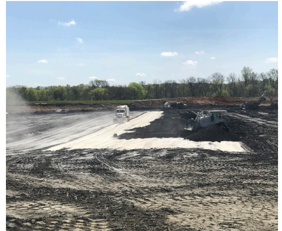
Lime Fines being spread by a Spreader Truck
