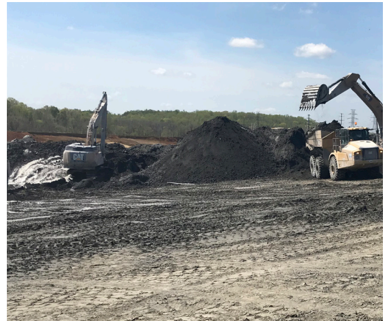
Pebble Lime being mixed in the Ash by an Excavator
