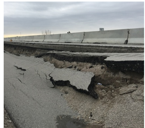
Pavement Slip Westbound SR 2 Ramp at SR 269 Ramp
